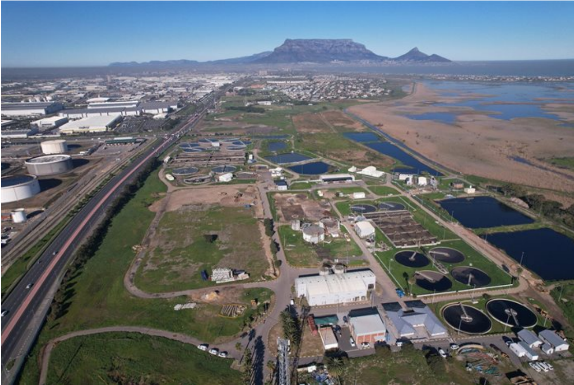
Potsdam Wastewater Treatment Works. Source: Supplied
